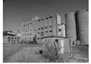
Shoreham Cement Works
